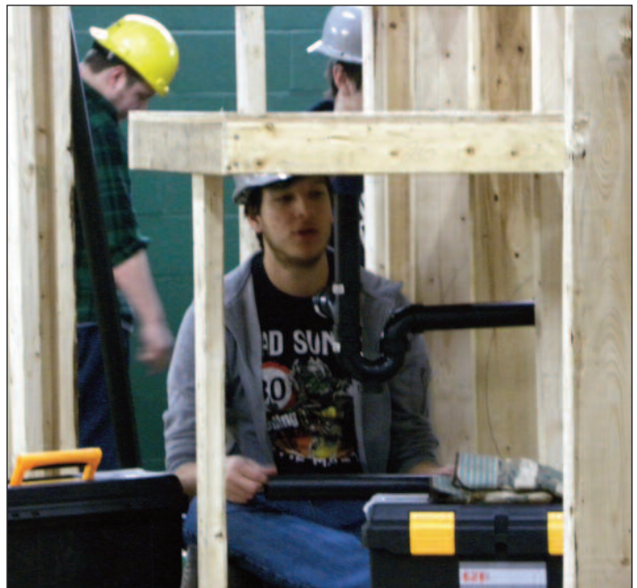
Verifying tail piece and P-trap are installed correctly. Below: Students in ITC advanced math class.
